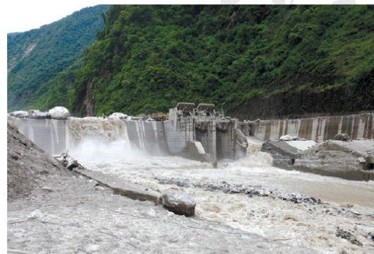
Bhotekashi Hydropower Dam on June 2016 Source: Uria News
